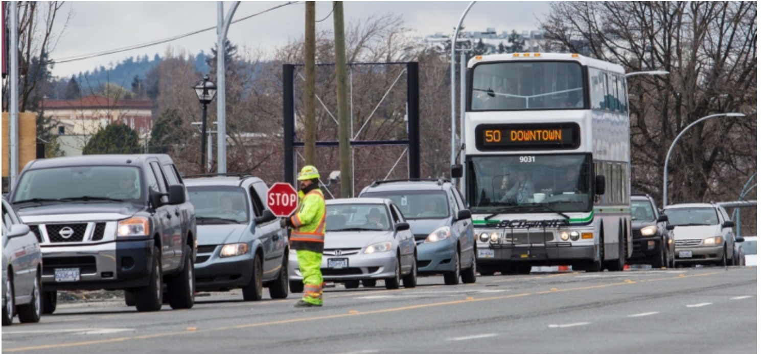
Traffic travelling through a construction zone along Douglas Street in Victoria.
